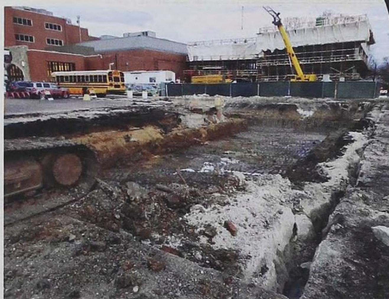
December 2019: As students left for Christmas break, construction workers dug a large hole in the existing parking lot so that a drainage system could be added.
